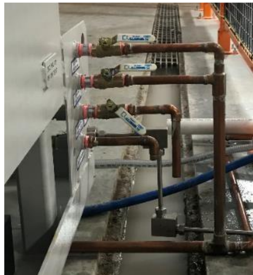
Figure 4 Water Connections Plumbed Example
