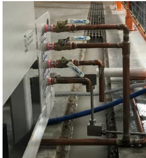
Figure 4 Water Connections Plumbed Example
