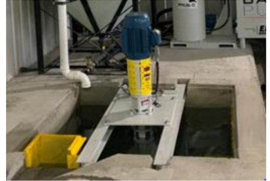
Keeping the pit pump ABOVE the water pit allows for the pump to be a more reliable and robust solution to draw the water out of the pit and into the recycling system rather than using a submersible pump which has the tendency to regularly fail by keeping it under water.
